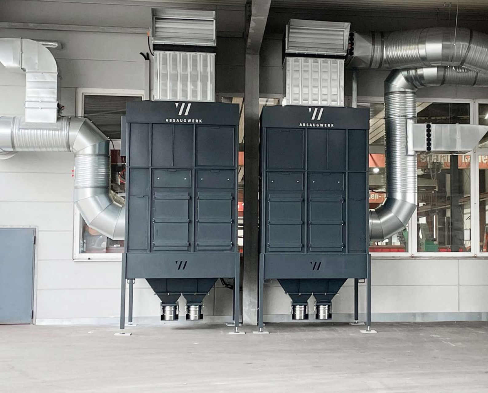
Series 7000 fume filters, 2-pack each with 37 kW of power
