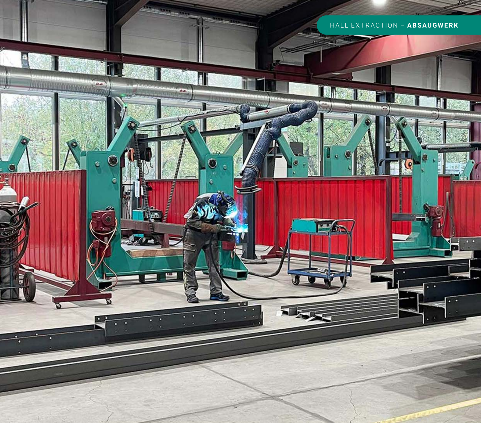
Direct extraction via extraction arms in combination with central hall extraction
