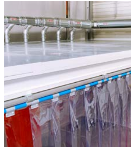
PIPE CONNECTIONS FROM THE BOOTH TO THE EXTRACTION SYSTEM
