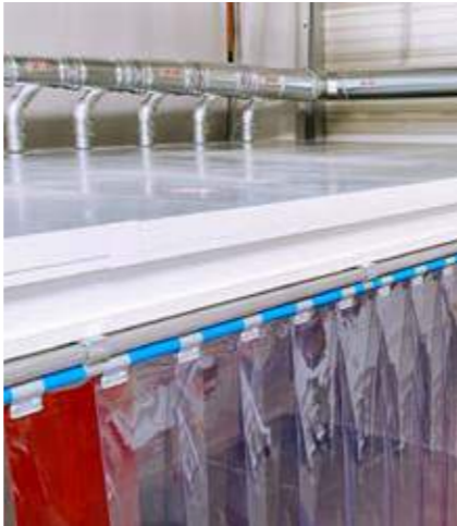
PIPE CONNECTIONS FROM THE BOOTH TO THE EXTRACTION SYSTEM
